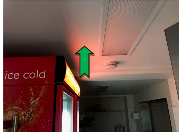
Photo 2. Interior, ground level, throughout, ceiling – non asbestos-containing fibre cement sheeting.
